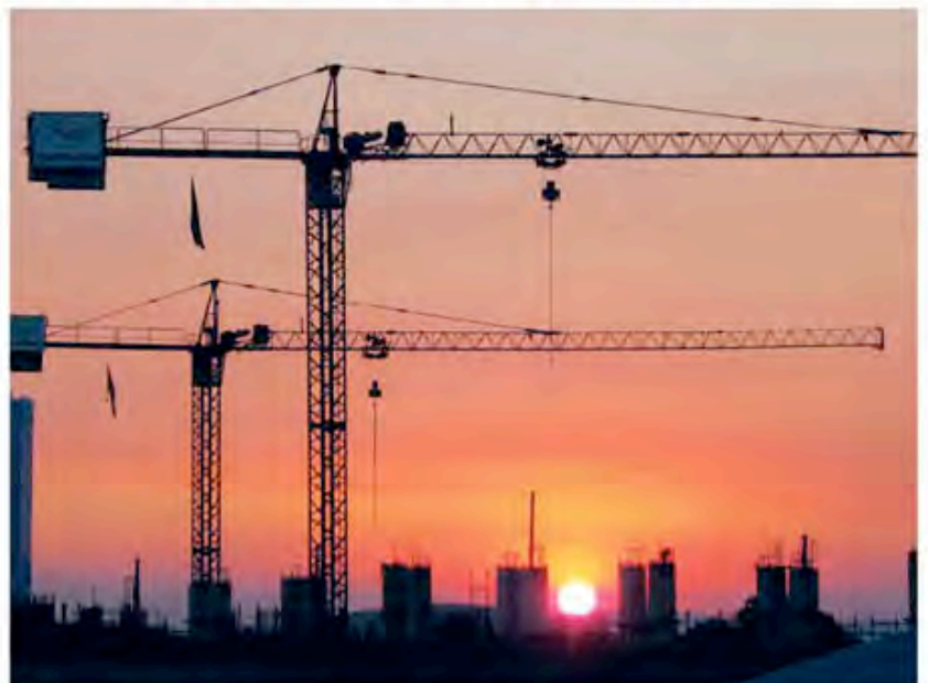
View of the Science Stadium under construction
